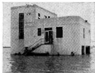
WWL's flooded transmitter
